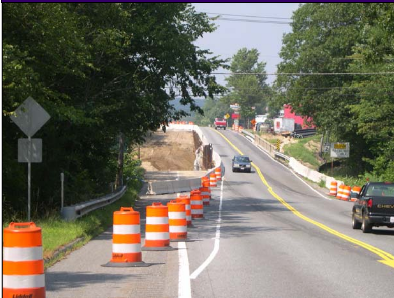
Reconstruction of Route 2 bridges in Ervingside.
