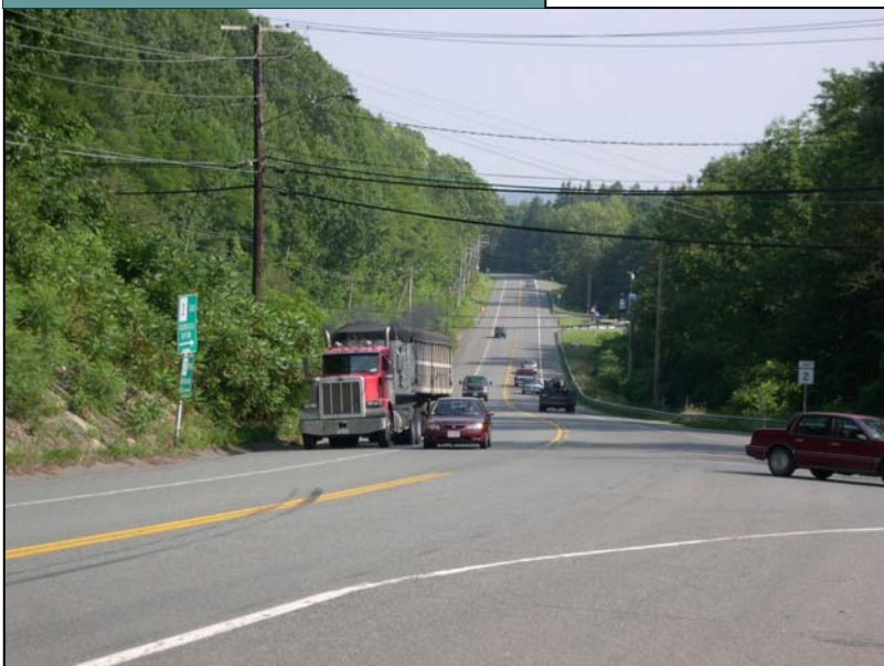
Difficult turns from Route 2 into Shelburne Falls addressed by the Road Safety Audit.
