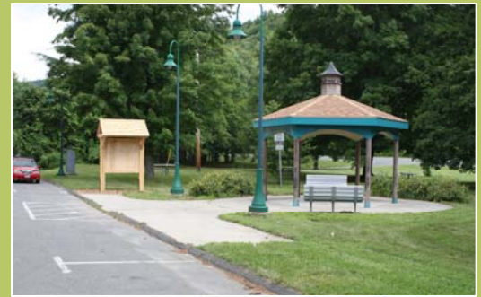
New Kiosk installed at the Shunpike Rest Area in West Charlemont
