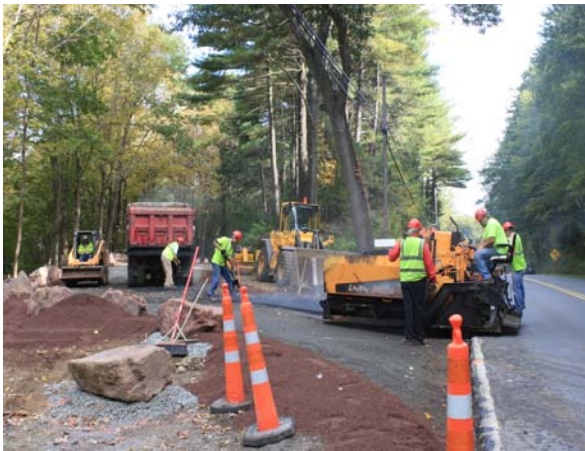
Construction Underway at the Sunderland Scenic Turnout Area
