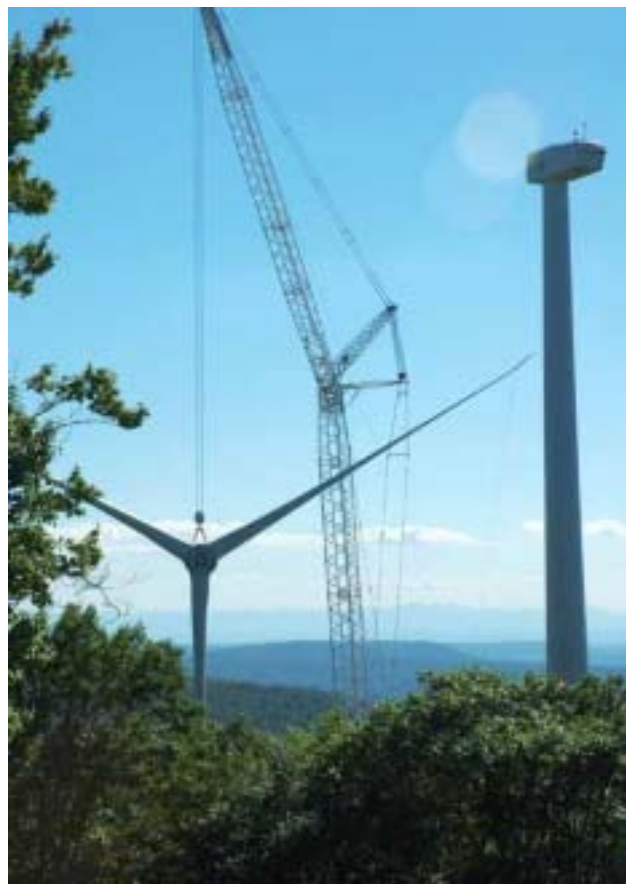
Wind turbine installation, Jiminy Peak-Berkshire Co.
