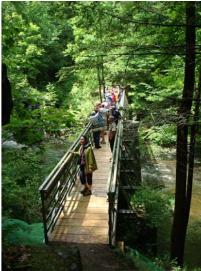
A view of the new pedestrian bridge that was installed over the South River on the Mahican-Mohawk Trail in Conway (photo credit: Whitty Sanford)
