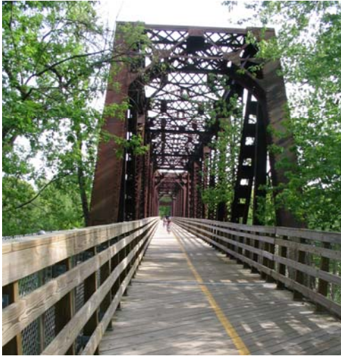
Former railroad bridge over the Connecticut River on the Canalside Trail
