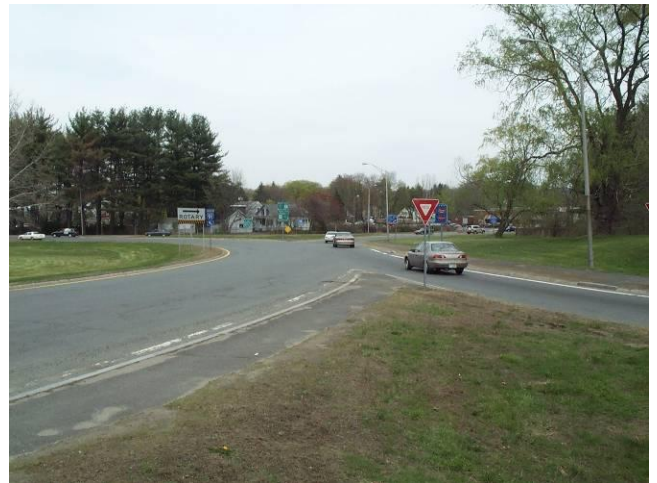
The Greenfield Rotary, prior to the implementation of safety improvements
