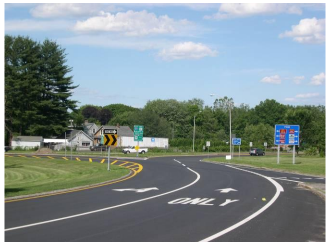
The Greenfield Rotary, after the implementation of safety improvements
