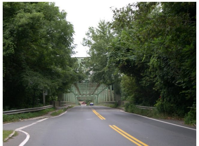
View of the General Pierce Bridge
