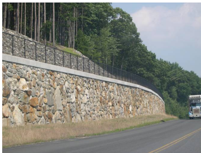
New retaining wall along Route 2, in Erving
